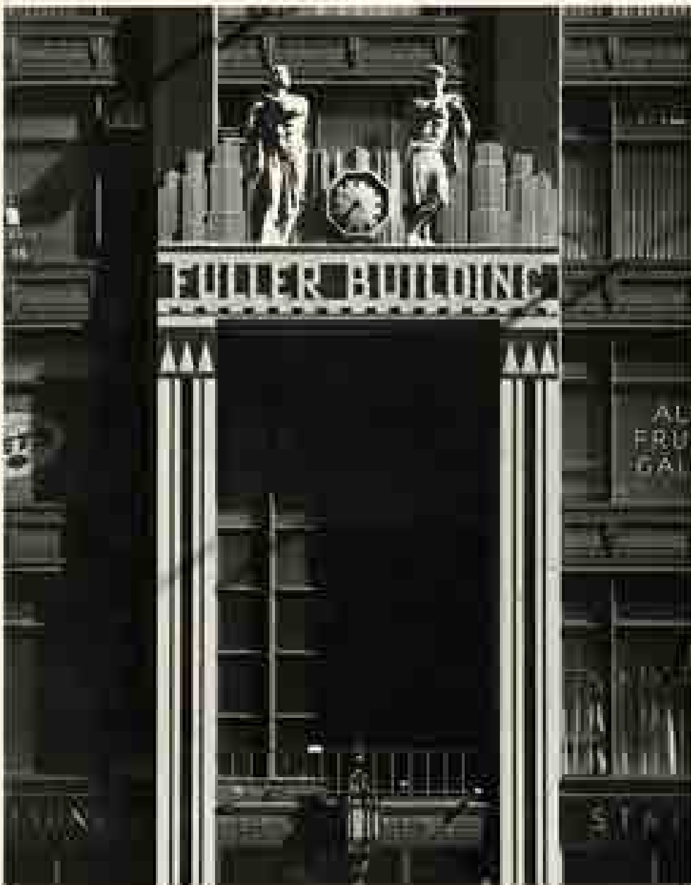
Fig. 4 Walker & Gillette, Fuller Building, 1928–29. Detail of the entrance.
